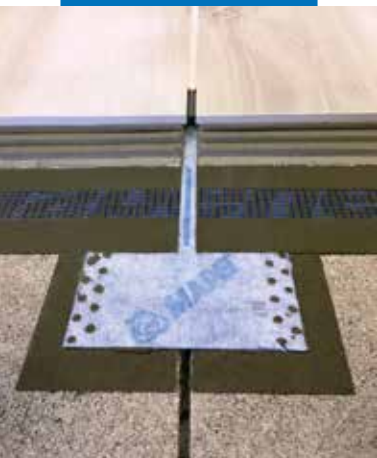
Mapeband Easy applied around a check-joint in the screed
