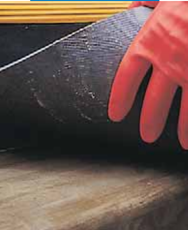
Installing rubber flooring on stairs with Adesilex LP
