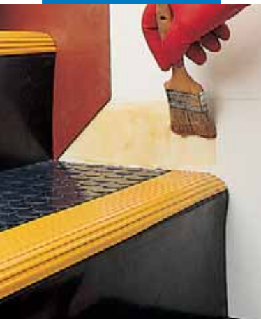
Installing rubber skirting with Adesilex LP
